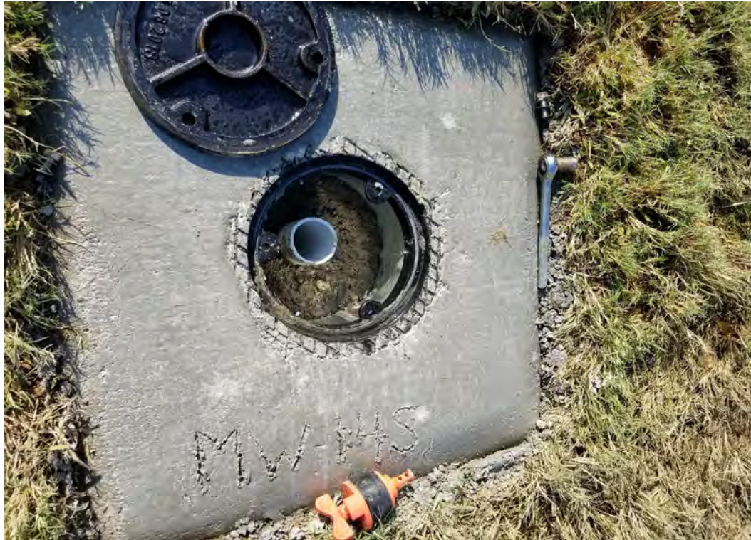
New Monitoring Well MW-14S
