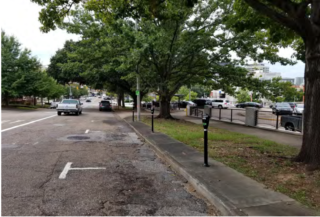
Washington Avenue Environmental Covenant (Facing West)
