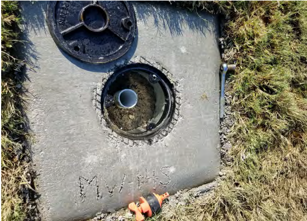
New Monitoring Well MW-14S
