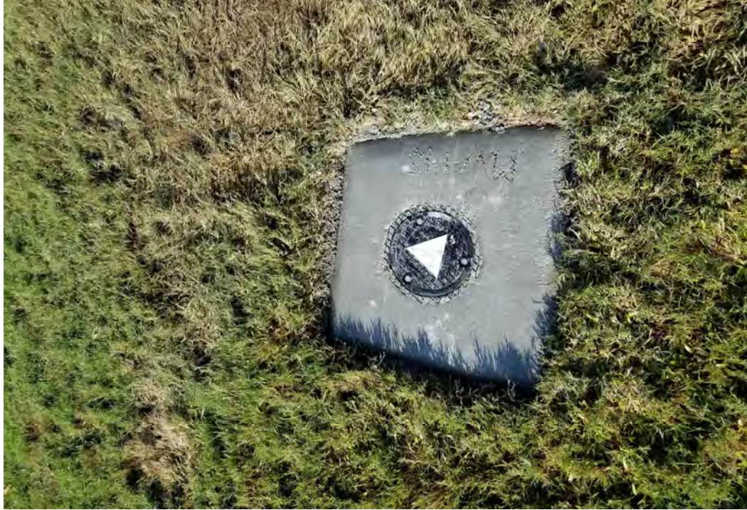
New Monitoring Well MW-14S
