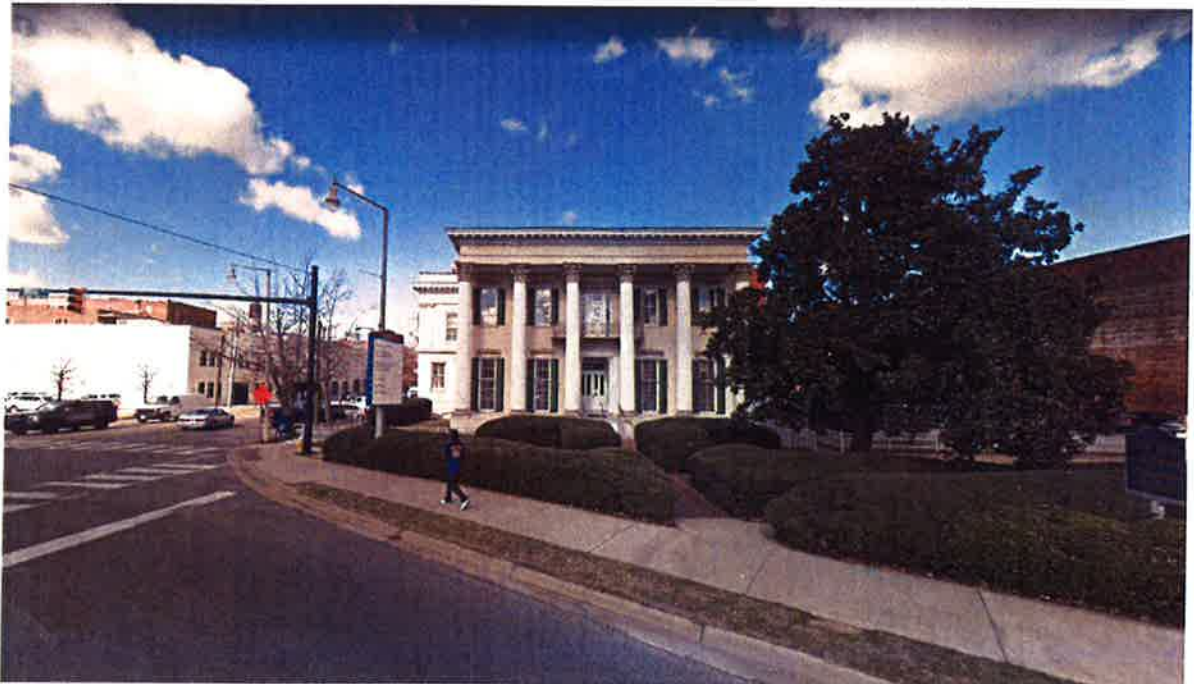
9. Surrounding buildings at Bibb Street
