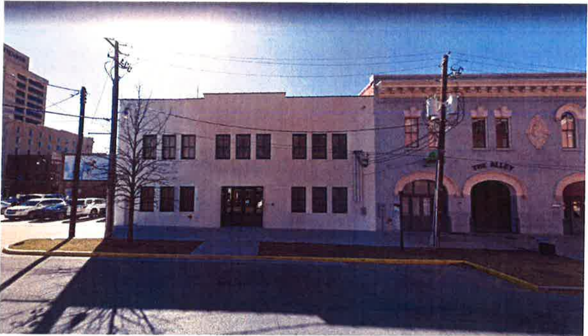
4. Surrounding buildings at Coosa Street
