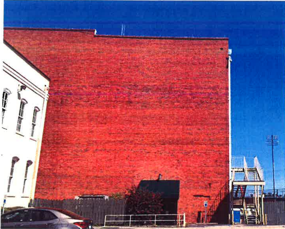
2. South elevation at Bibb Street
