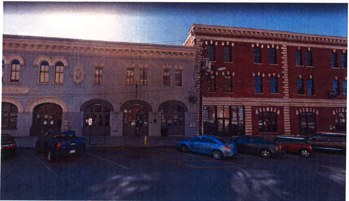
5. Surrounding buildings at Coosa Street
