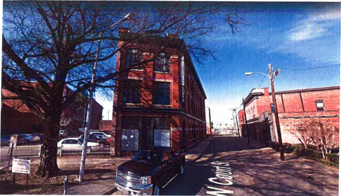
8. Surrounding buildings at N Court Street
