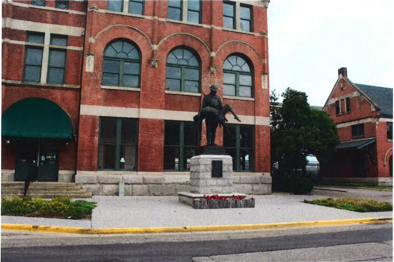
Previous installation in front of east block, plinths to match in style (not size)
