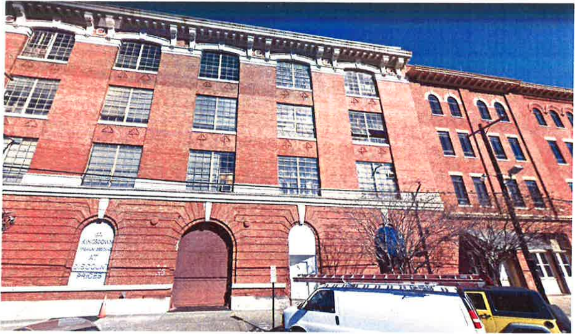
6. Surrounding buildings at Coosa Street
