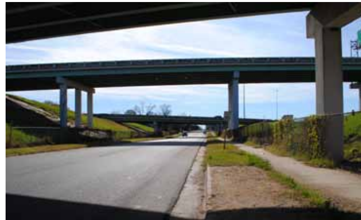
Figure 6: Current pedestrian experience at the Interstate interchange above Holt Street looking south.
