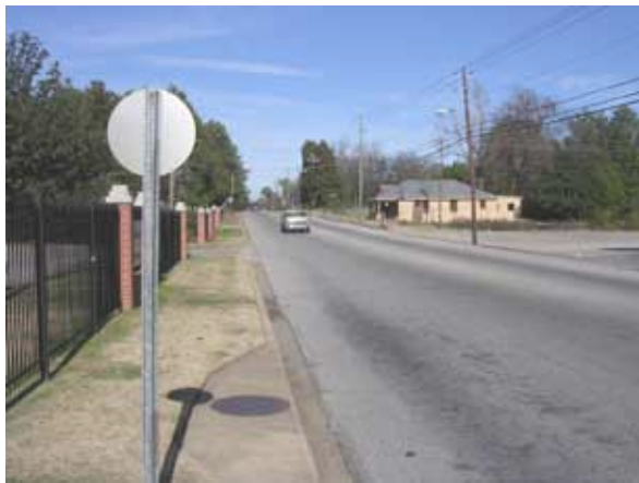
Figure 27: Existing conditions along Holt Street near St. Jude.
