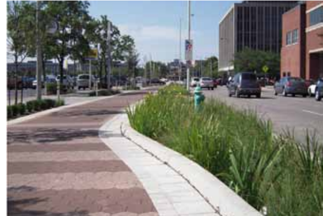
Figure 59: Rain garden along the trail. Used with permission from Indianapolis Cultural Trail, Inc.
