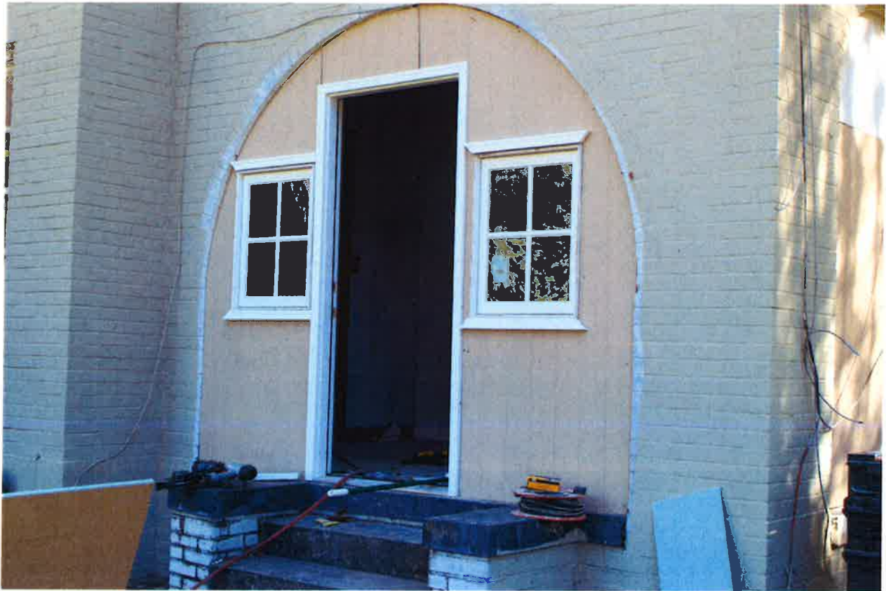
3179 Norman Bridge Road
