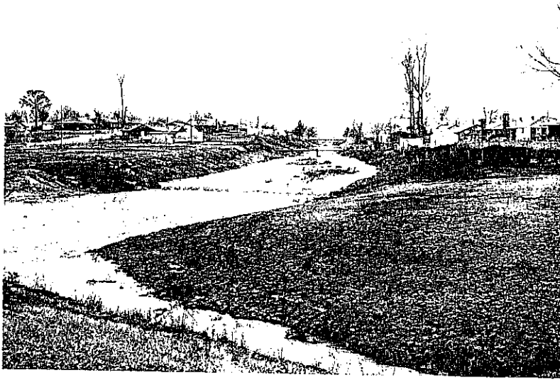
FIGURE 2-1. Natural drainage channel through a subdivision near Lagoon Park (note the check dam).
