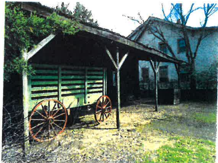
Front shed view
