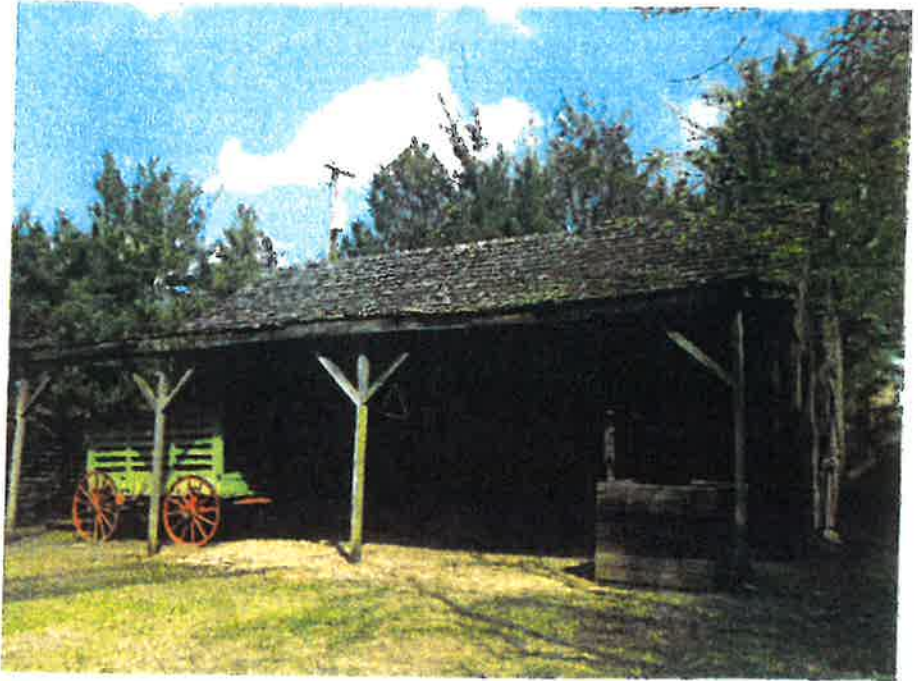
Front shed view
