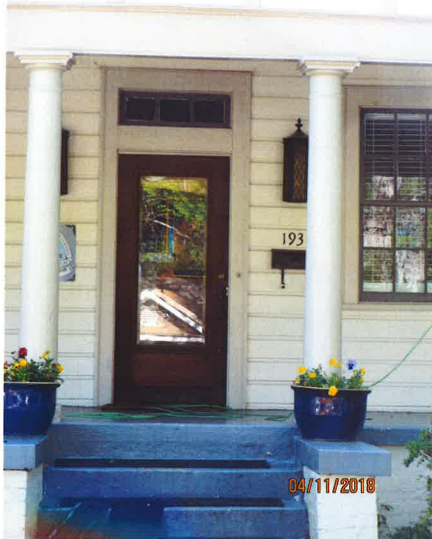
Door across the street—glass with beveled edge and stain finish. Appears original.
