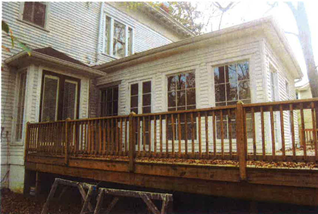
Current West Elevation (previous addition)
