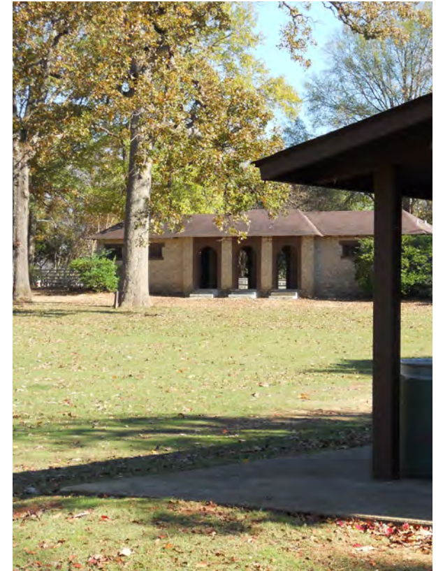
Oak Park picnic shelter and main building
